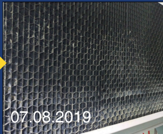
As a result of comparison before and after the operation of the cooling tower eliminator in the bottled water plant in Korea, it can be seen that the scale of the surface was removed 35 days after operation
